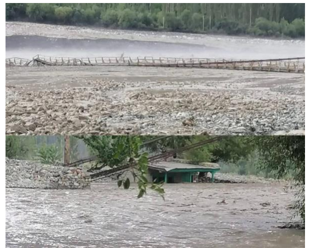
Figure 11 Asia's longest suspension bridge destroyed by flood
